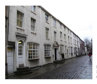
Fig.12: Numbers 15 and 17 Wood Street have been rendered but retain some original details.
