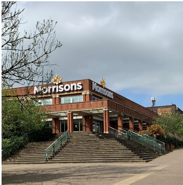
Figure 1: Morrisons Superstore occupies the former Atlas Mills site, presents a prominent and well-established anchor presence and mobility-impaired pedestrian access from Mornington Road level.
