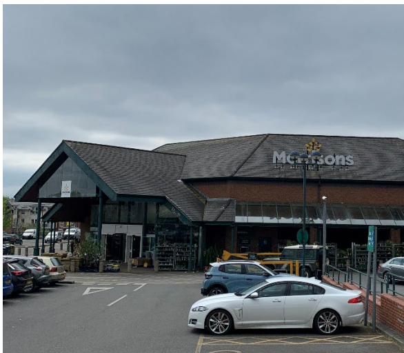
Figure 1: The Morrisons Superstore presents a well-maintained, pitched-roof suburban format with active frontage, accessible car parking including dedicated disabled bays.
