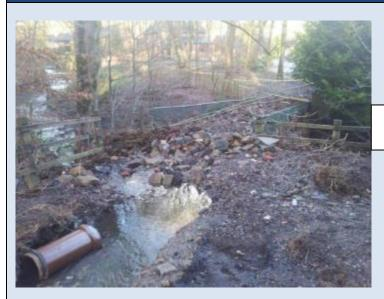
Landslip debris and damage to footbridge
