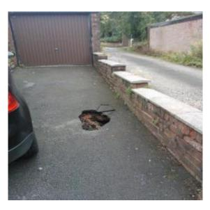
Picture 2 Hole appeared due to Pickhill Brook culvert collapse below
