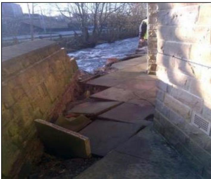
Picture 1 Collapsed section of flood wall at Littleborough
