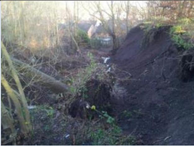
Land Slip showing land eroded by culvert collapse
