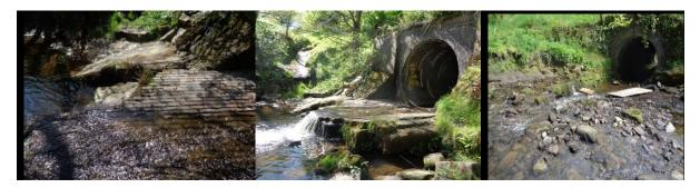
A feasibility study was undertaken, and a scheme designed to secure the failing culvert. The works included grouting the culvert anulus, replacing the training walls, refurbishment of the retaining walls, replacement of the highway drainage and to prevent further downstream movement, a new spillway installed that includes piled reinforcement.
