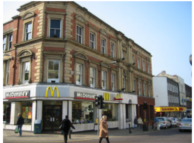
McDonalds Restaurant on the south east corner of the St Helena area
