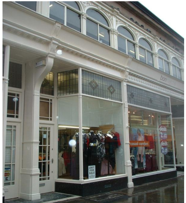
The Market Hall in Bolton. This traditional shop front displays all the basic components of shop front design and follow a consistent design, which provides an attractive frontage to the Market Hall
