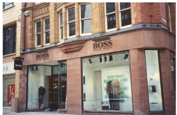
'Less is more' The stone fascia and pilasters of the building above create a distinctive surround that frames the large glazed openings. Applied bronze lettering adds subtle and effective advertising.
