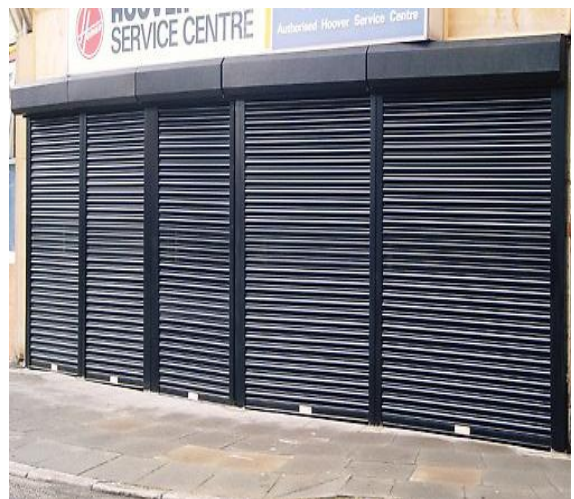
Solid Security Shutters, which cover the entire shop frontage are not acceptable
