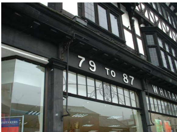
Division of glazing with framing adds visual interest and breaks down the scale of the shop front
