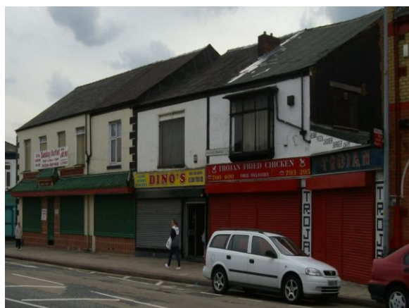
Solid external roller shutters provide a dead, unattractive frontage
